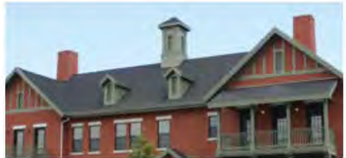
Roof Materials: Asphalt Composite Shingles
