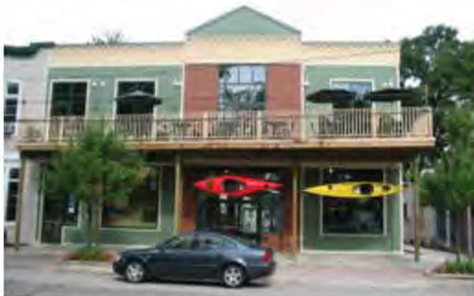
Primary Materials: Painted Wood
