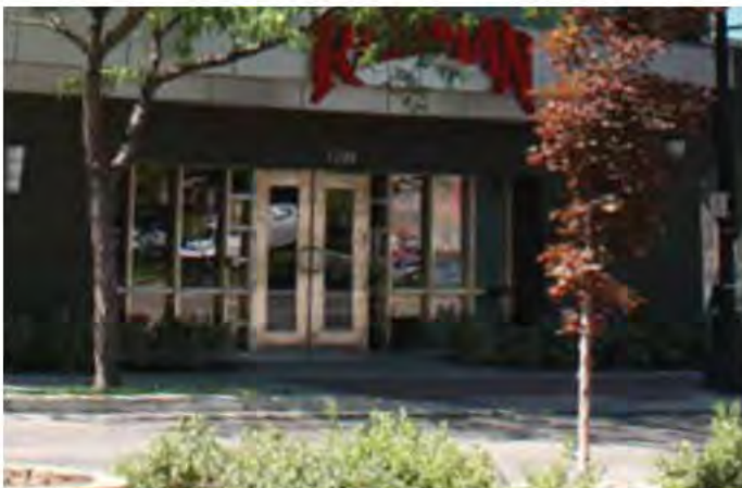
Permitted: Commercial Grade Doors & Windows on Commercial Buildings
