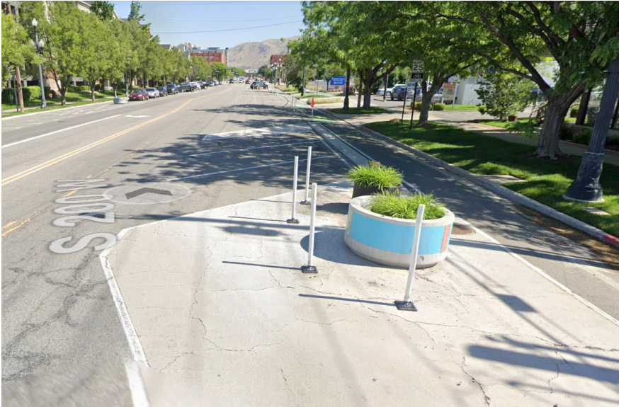
In SLC, 200 W was reconfigured with protected bike lanes using simple materials
