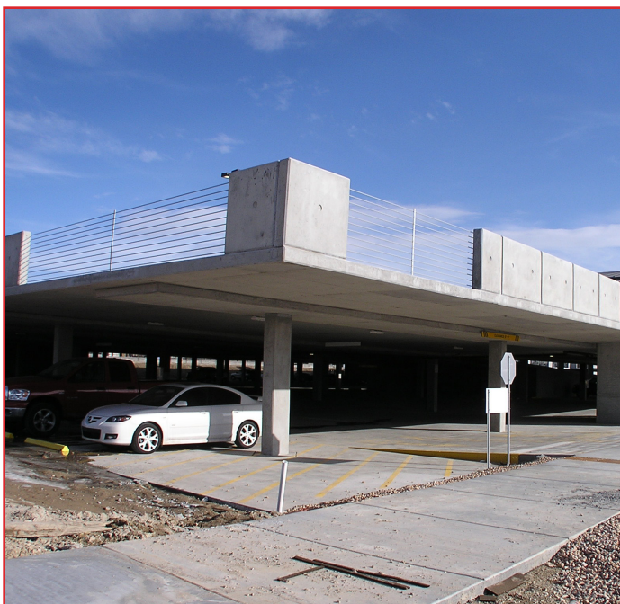
Park and ride parking garage
