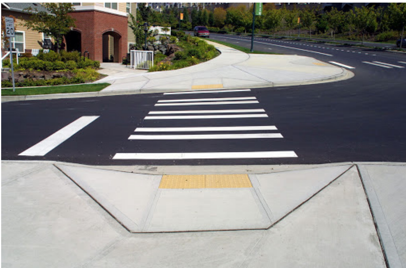
Safe ADA compliant crosswalk
