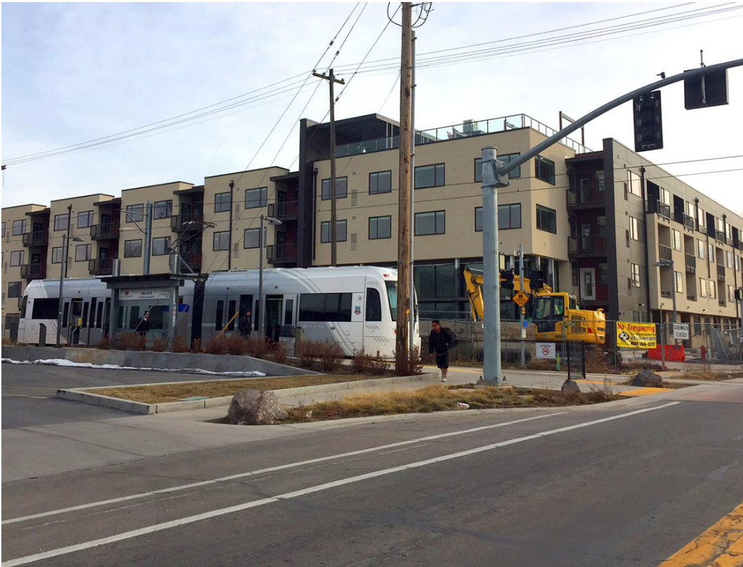
Increasing the level of density around transit service makes the service more viable
