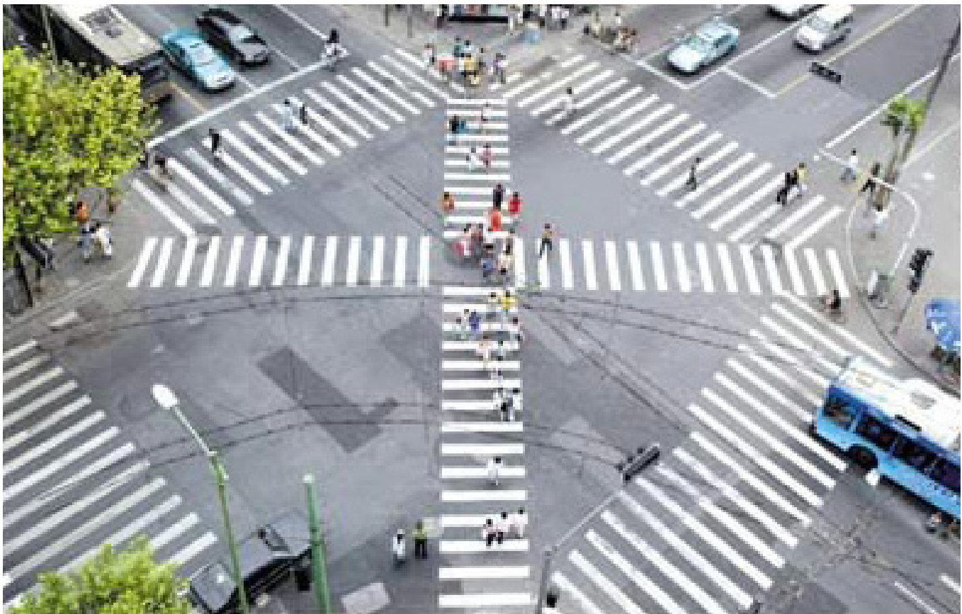
Diagonal crossings improve pedestrian route safety and efficiency by minimizing the time spent at and within intersections
