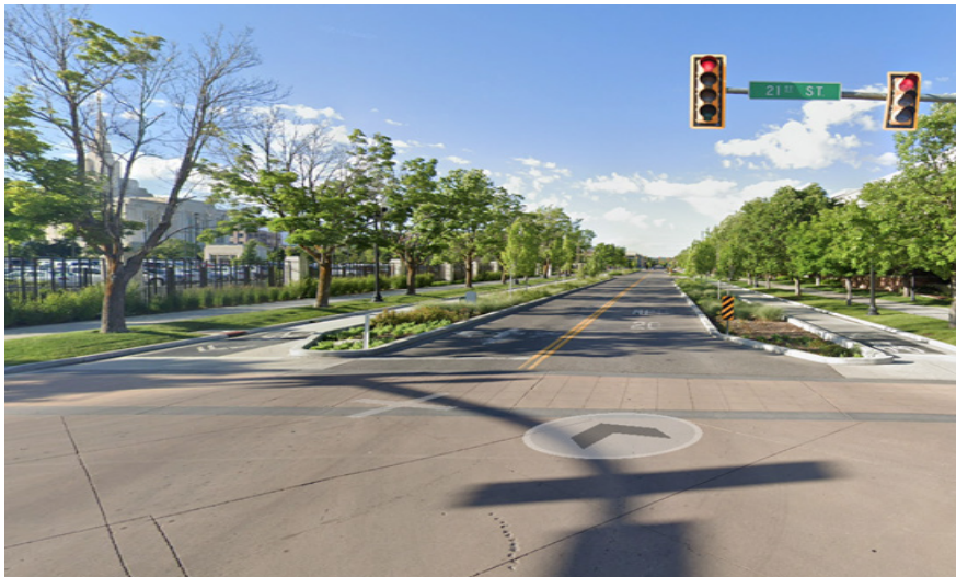
Landscaped barriers are used for protected bike lanes.
