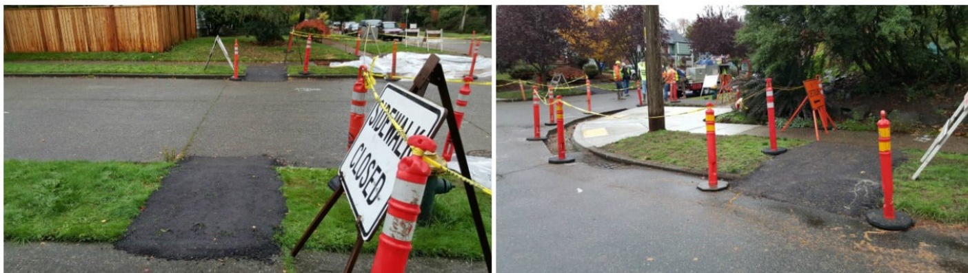
Temporary ADA-compliant connections should be created for pedestrian and bicycle paths during construction.
