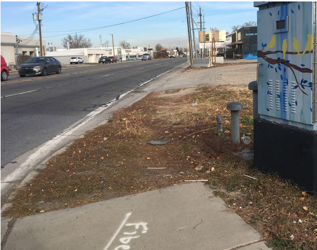
Discontinuous sidewalk in City of South Salt Lake
