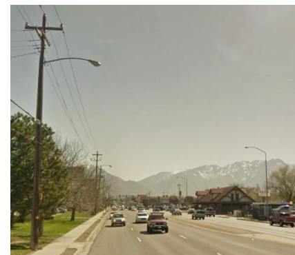
Lights Mounted to Power Poles where conflict exists.
